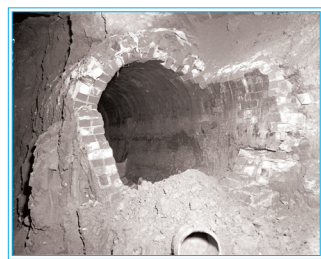
Old Sewer under Front Street
